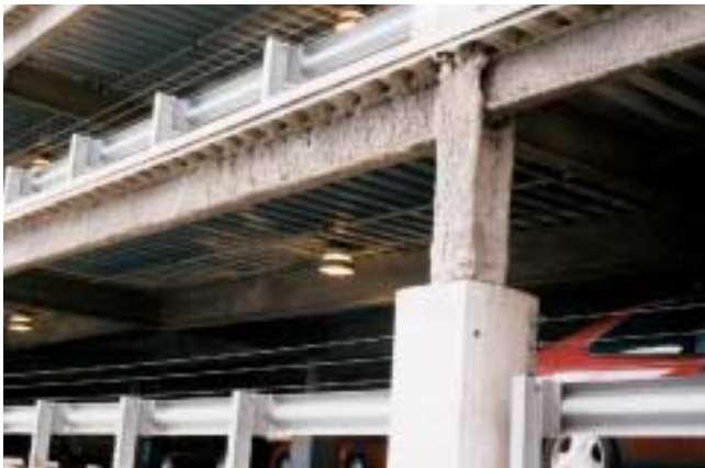
Figure 13-13 This parking garage is of Type II construction. The protective coating applied to the structural steel may increase the fire-resistive rating, but note that the unprotected corrugated metal flooring and interior steel structure are not protected. These unprotected structural members may fail early in a fire. (Photo courtesy of William H. Schmitt, Jr.)
