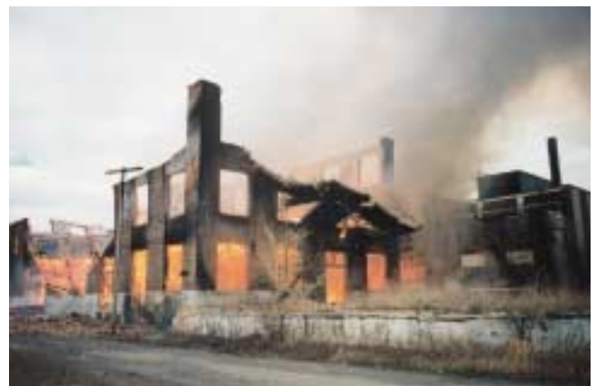
Figure 13-36 These photos show the effects of fire on a masonry wall. Note the debris and distance the bricks fell away from the building. Firefighters should always establish a collapse zone, as shown in Figure 13-35.
