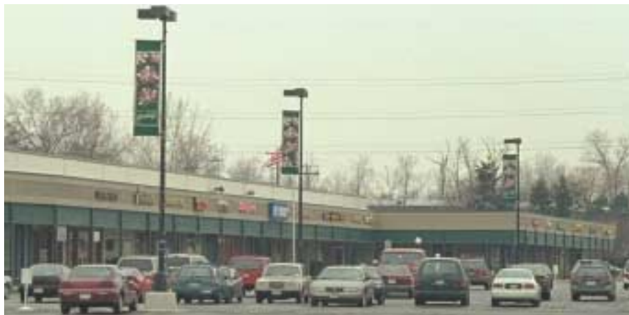
Figure 13-18 One of the most common uses of Type III, ordinary construction, is the “strip mall” with masonry walls and lightweight steel or wood trusses. Common problems associated with this type of construction are void spaces allowing for rapid fire extension and collapse of lightweight structural elements.
