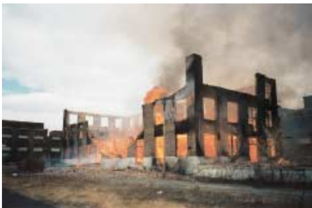
Figure 13-36 These photos show the effects of fire on a masonry wall. Note the debris and distance the bricks fell away from the building. Firefighters should always establish a collapse zone, as shown in Figure 13-35.
