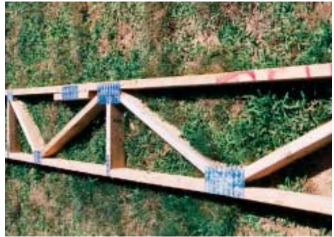
Figure 13-27 A typical parallel chord truss. The gusset plates on this truss are pressed into the wood. In addition to the decomposing of the wood element, the light-gauge steel plates will deform and pull away from the wood under fire conditions.
