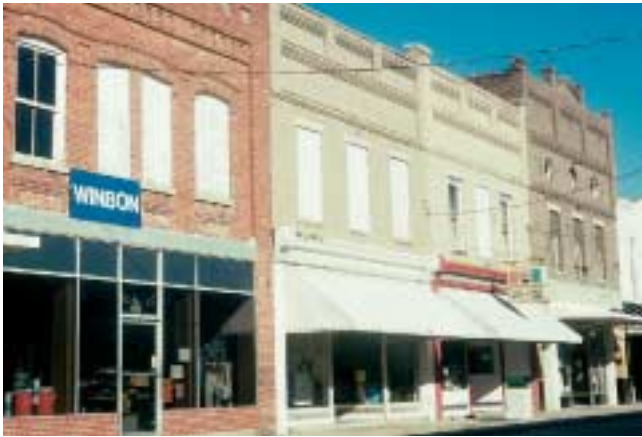
Figure 13-17 Buildings of Type III, ordinary construction, are common throughout North America. These typical “Downtown USA” buildings provide many challenges to firefighters, such as void spaces and common walls allowing rapid fire extension and little structural protection, with early collapse during firefighting operations.
