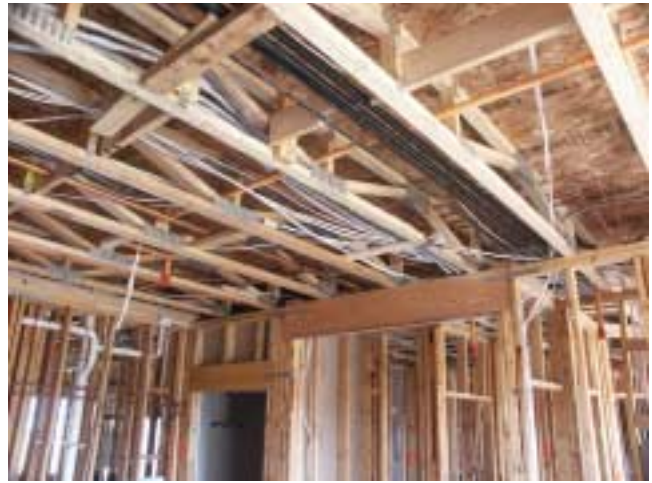
Figure 13-29 Lightweight floor truss systems have many void spaces. This could be called “horizontal balloon frame.”
