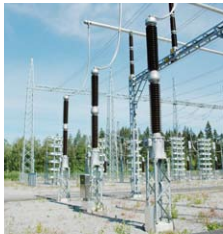
Capacitive voltage transformer ABB type CPA for 420 kV
