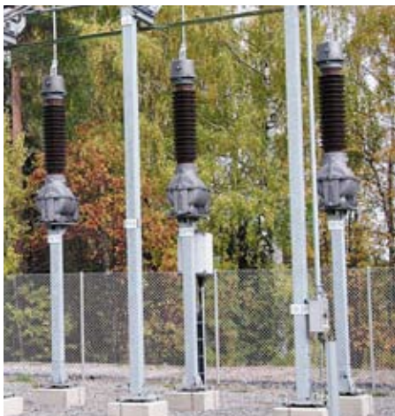
Inductive voltage transformer ABB type EMF for 145 kV
